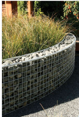
Short Gabion Wall
