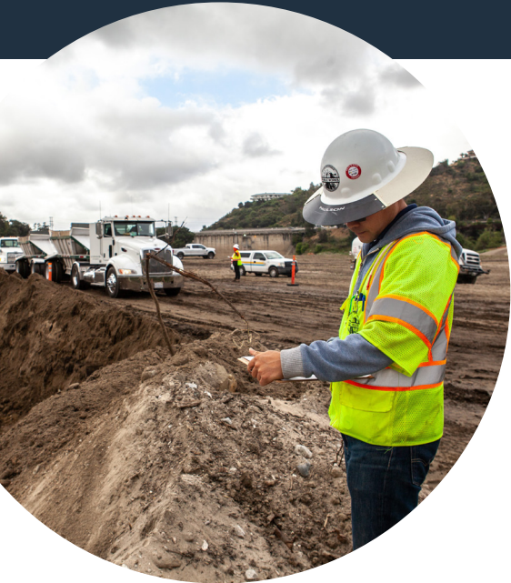
Public Works inspector hard at work on the job site.
