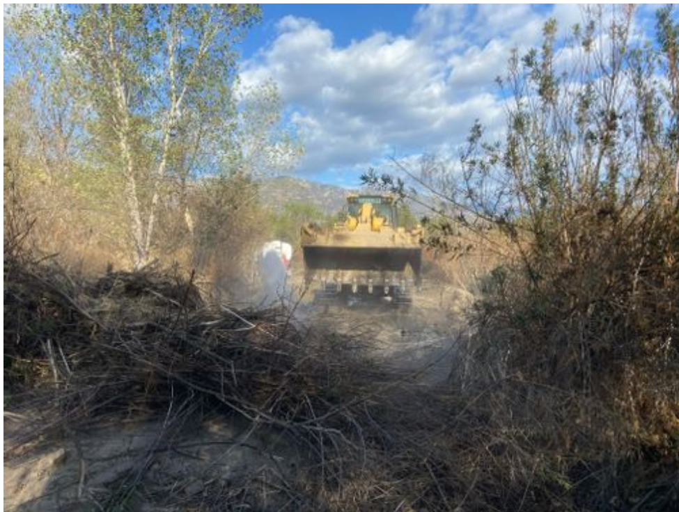
Vegetation clearing activities.jpg
