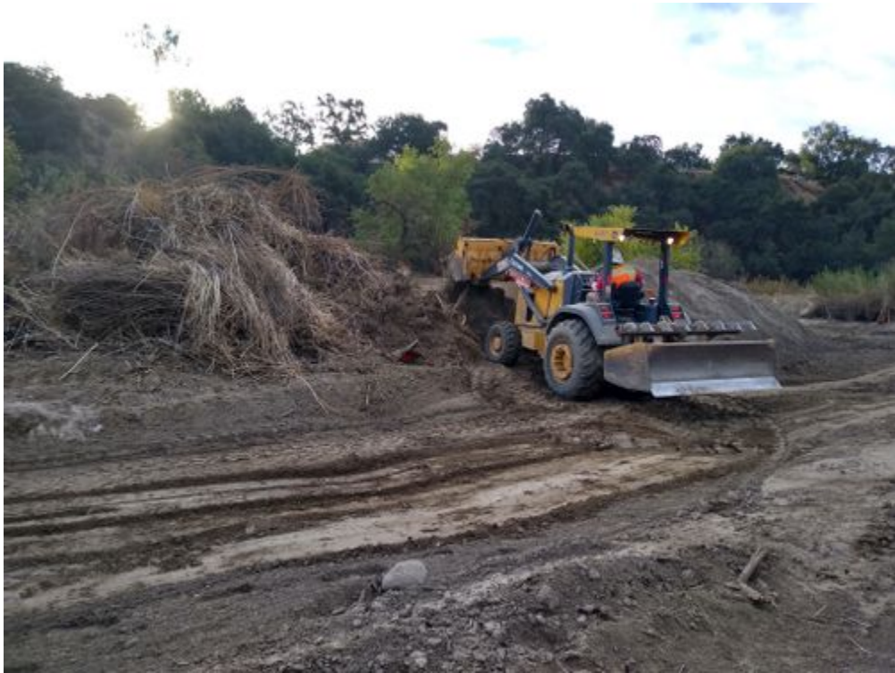
photo_2-skip removing vegetation pile.jpg -118.17203 34.19097
