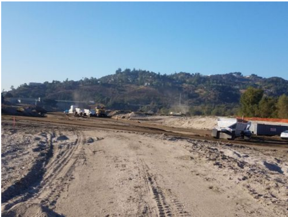
photo_2-20201113_sediment removal_facing S.jpg -118.1724 34.1922
