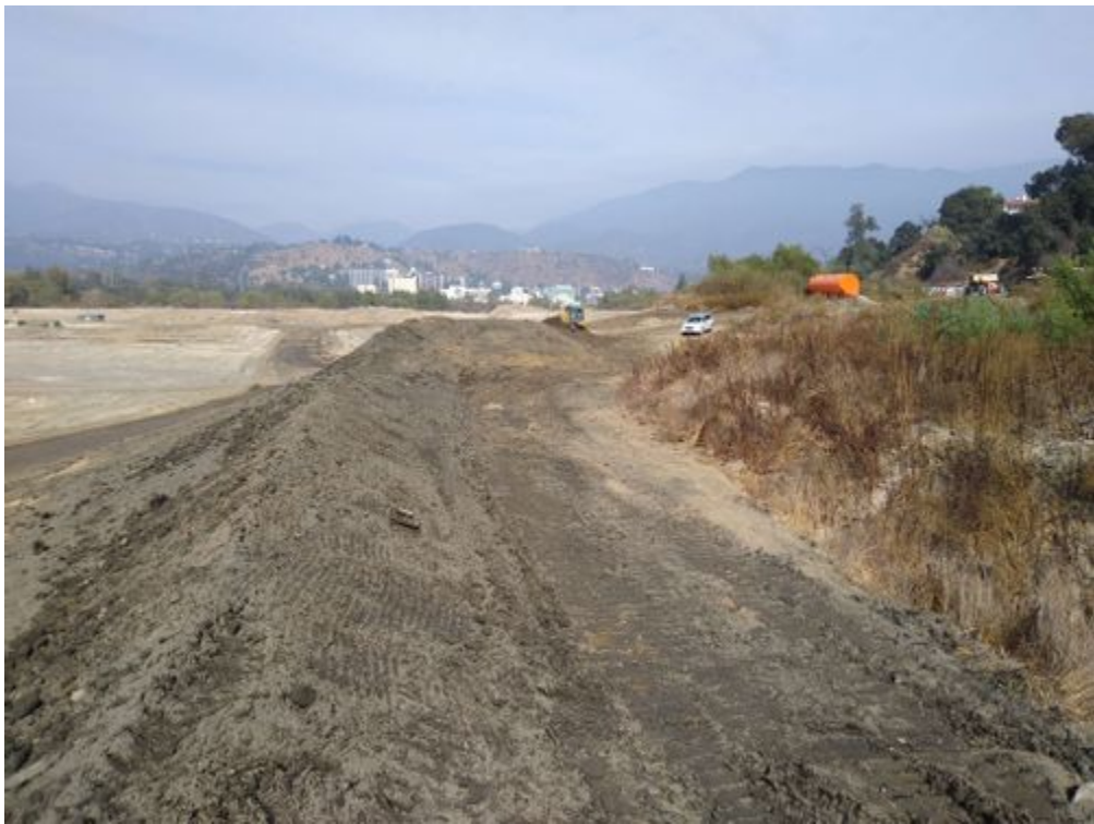
photo_2-rebuilt slope near Alta Dena drain.jpg -118.17347 34.18699
