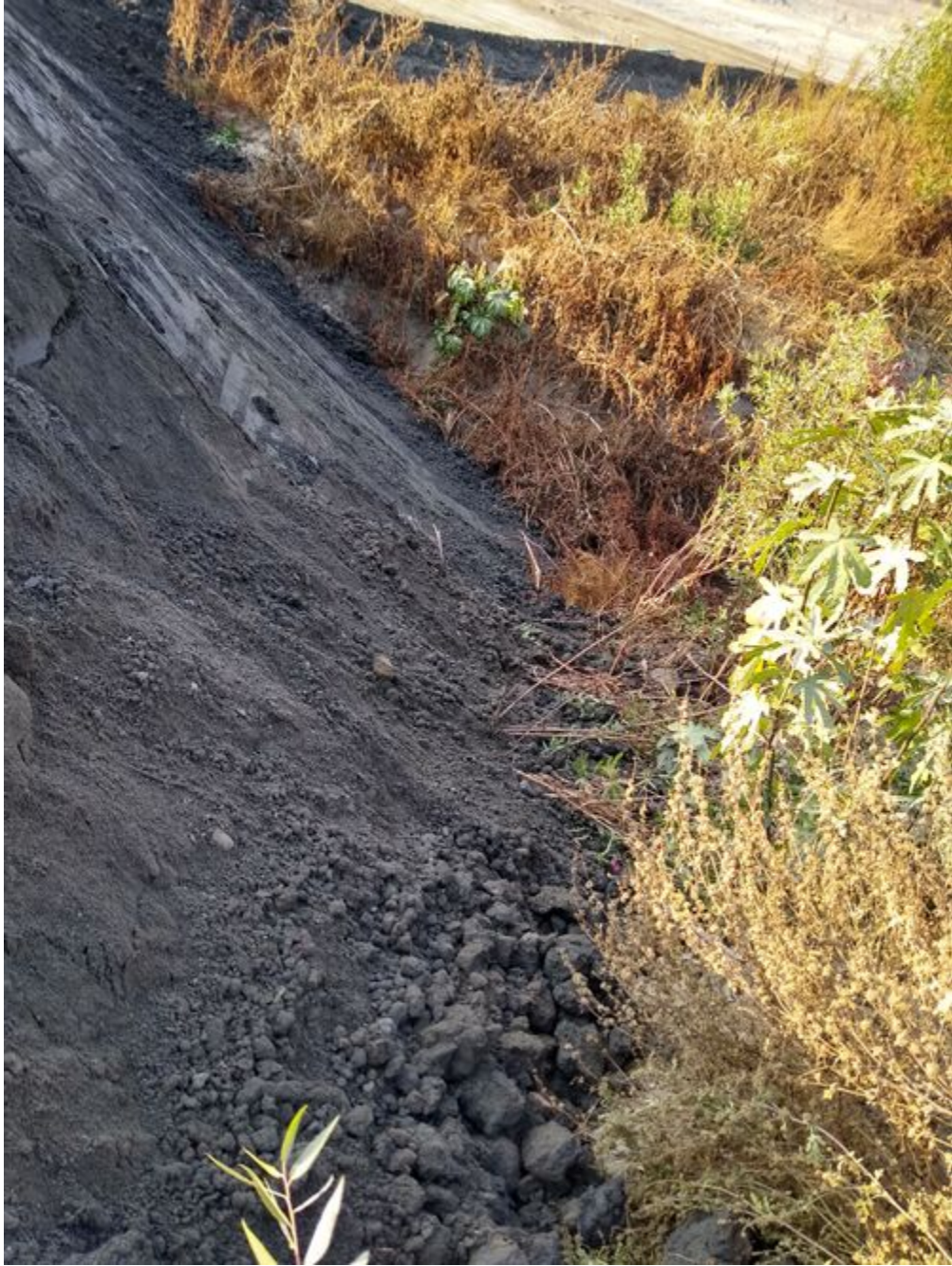
photo_3-area where irrigation affected.jpg -118.1734 34.18693
