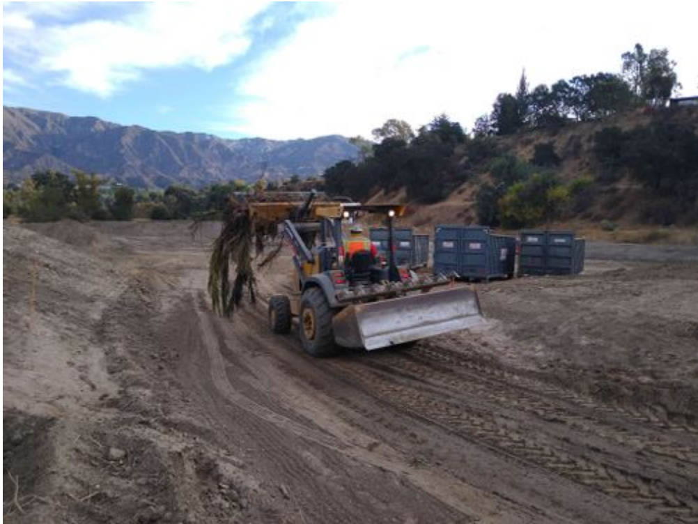
photo_1-skip removing vegetation stockpile.jpg -118.17205 34.19097
