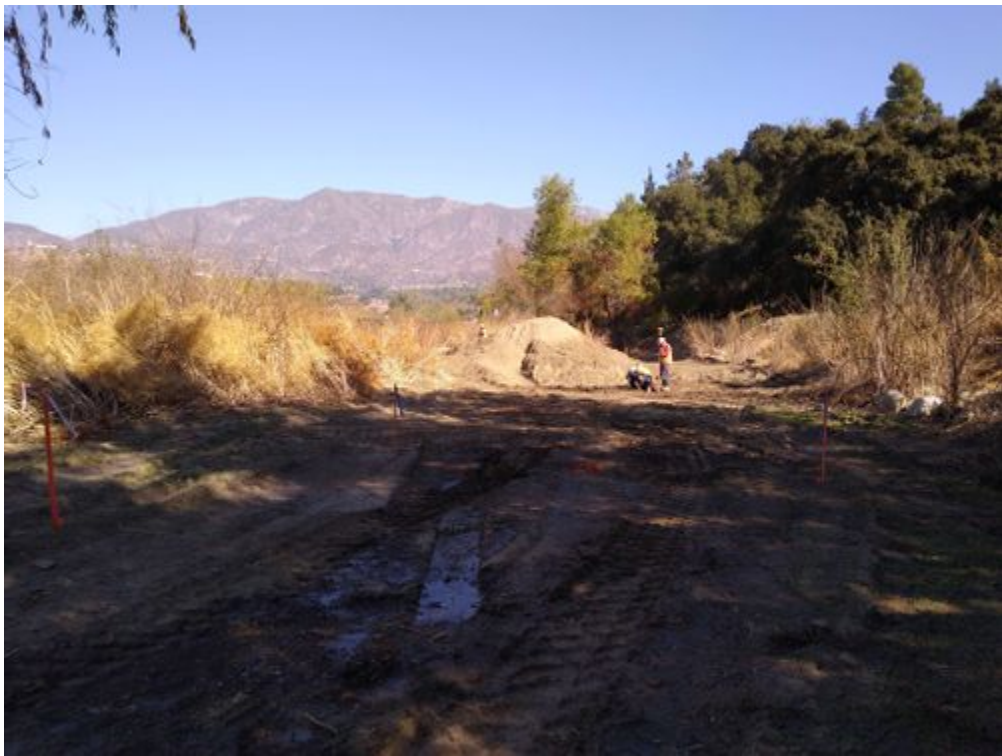
photo_2-dozor stockpiling fill.jpg -118.17208 34.18997
