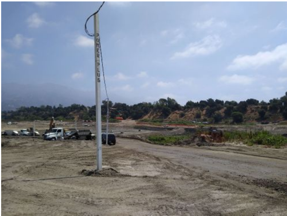
photo_2-sediment hauling activities.jpg -118.17644 34.18686
