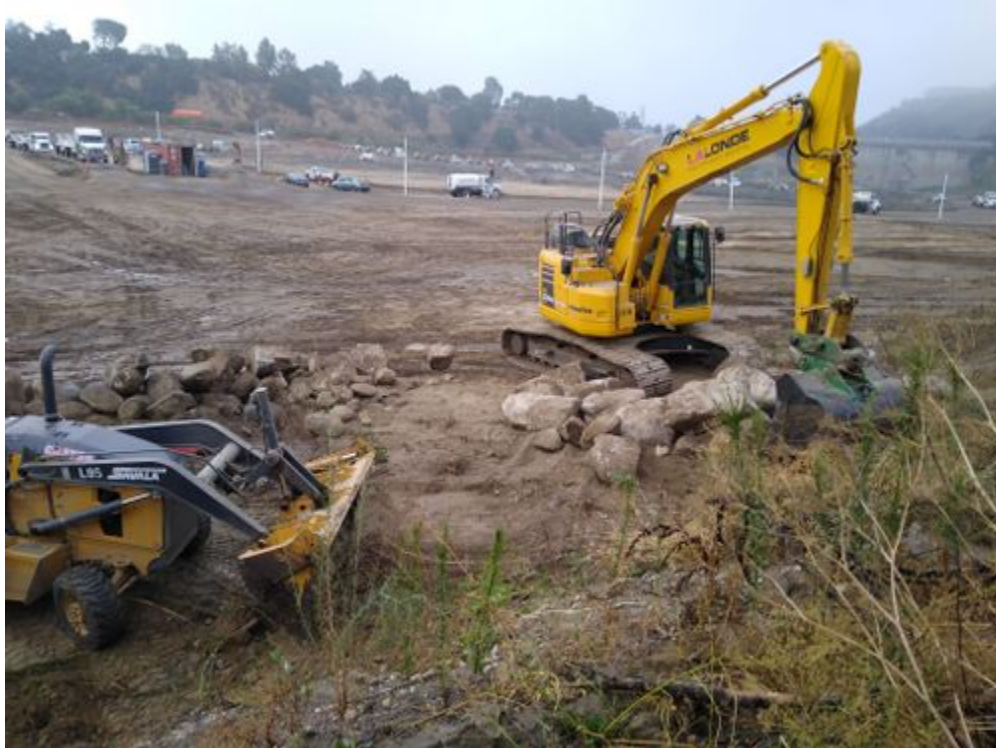
photo_1-excavator and skip moving boulders.jpg -118.17555 34.18966
