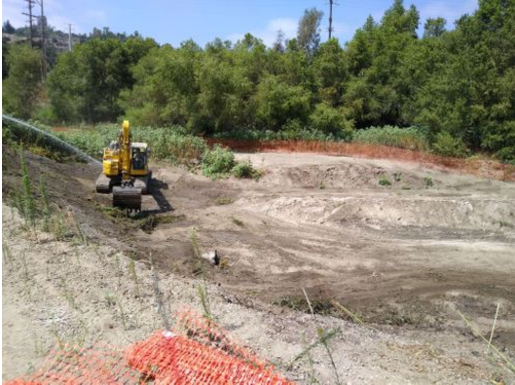
photo_1-excavator removing vegetation.jpg -118.17644 34.18685
