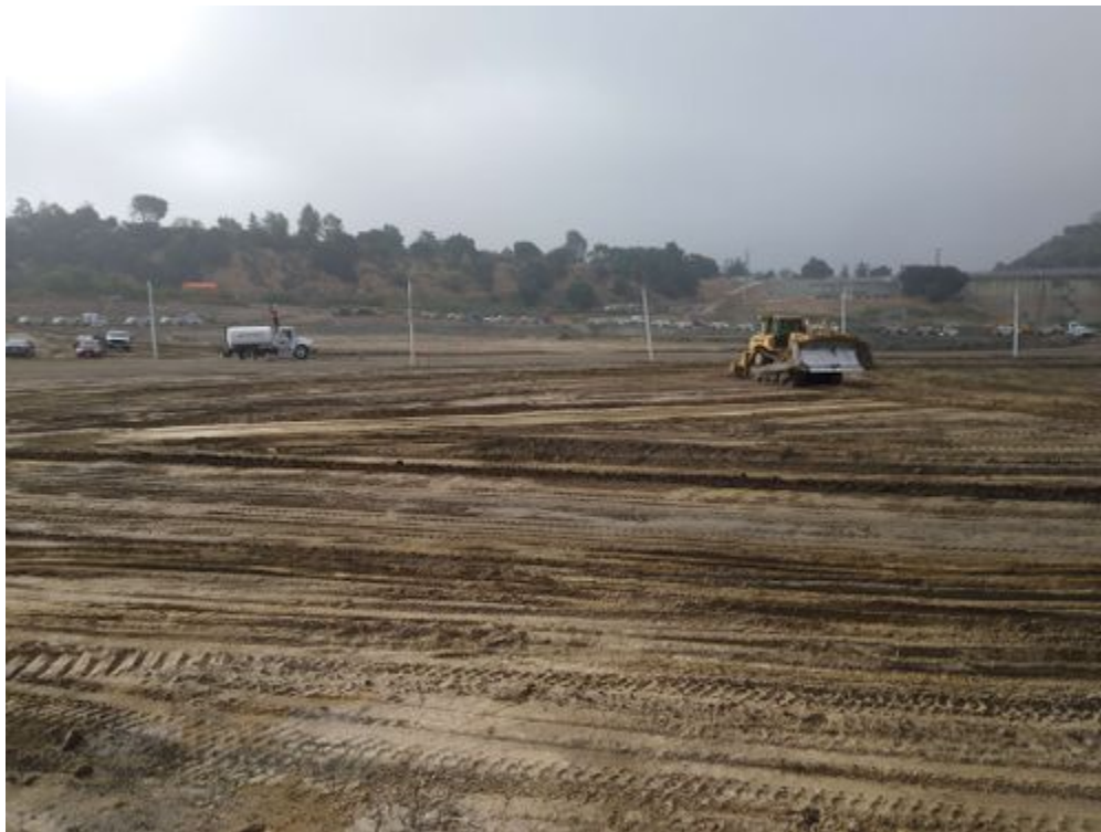
photo_2-sediment hauling activities.jpg -118.17565 34.18935
