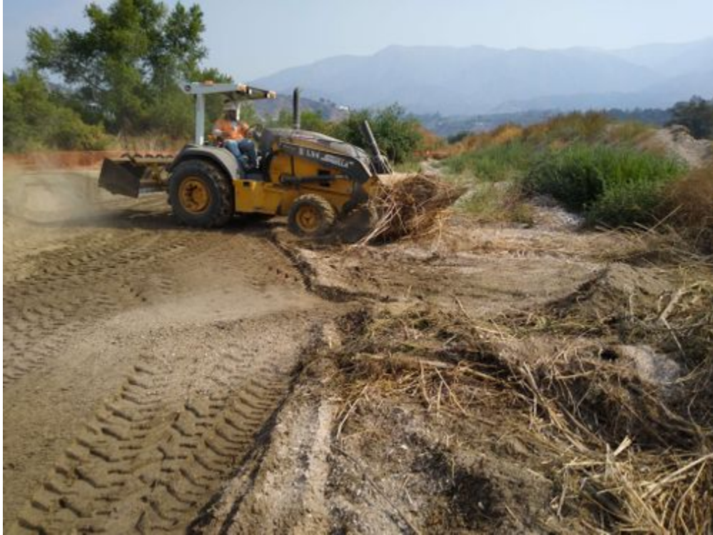
photo_1- vegetation removal.jpg -118.17272 34.19226
